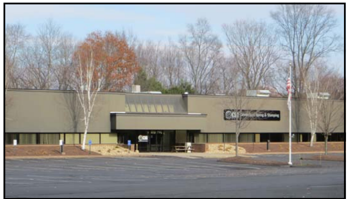
North Facility—51,000 Sq. Ft. 28 Spring Lane
